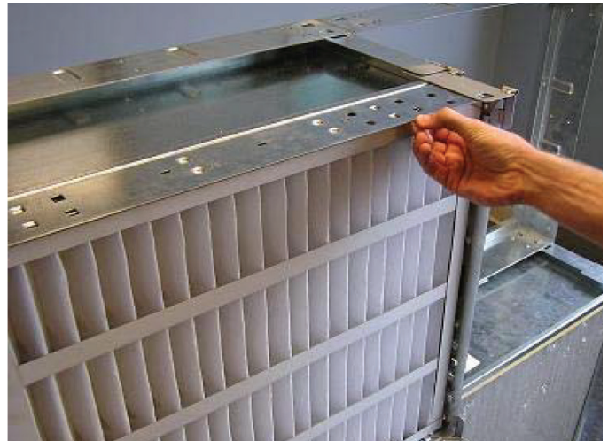
Figure 31: Installation of Prefilter into Frame
