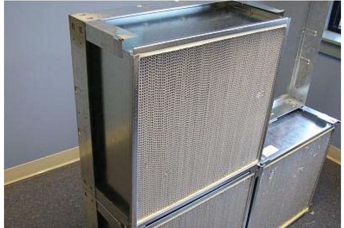
Figure 21: Filter Placed Inside of Frame
