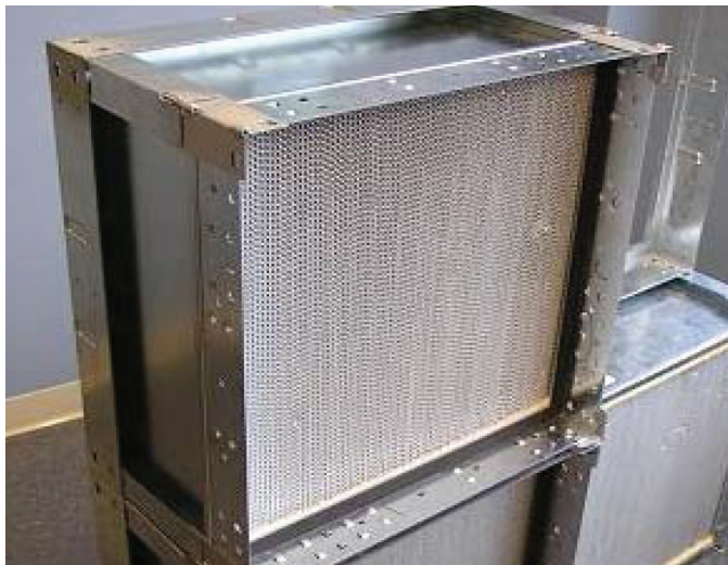
Figure 30: Properly Installed HEPA Filter
