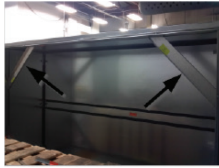
Figure 5: Shipping Braces
