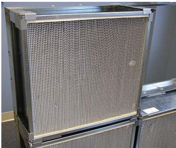
Figure 25: Properly Installed Filter Inside of the Frame
